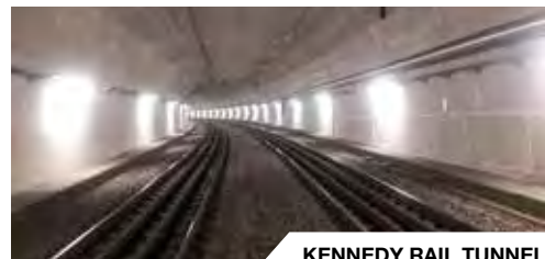
KENNEDY RAIL TUNNEL
