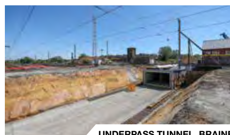
UNDERPASS TUNNEL, BRAINE
